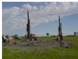
Well Field Drilling
